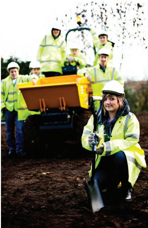
Young people working on the Donaldson Court (formerly known as Miller Road) project
