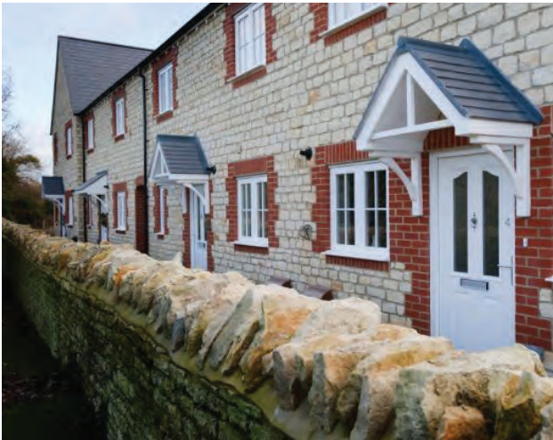
A rural exception site development at Bramley Close, Gosford which delivered 36 affordable homes
