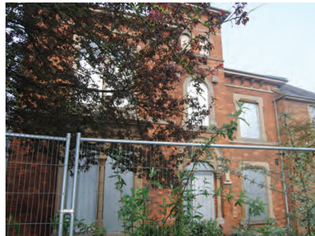
An empty property in Banbury that will be returned to use as part of CDC's "Build!" programme
